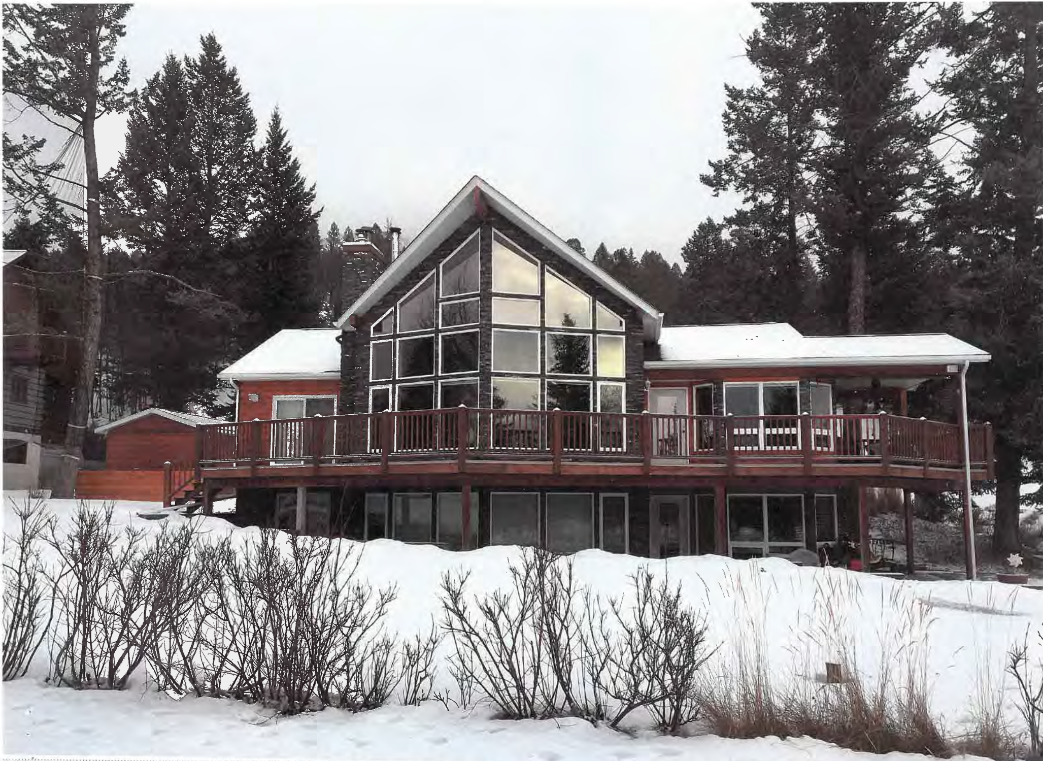
SUBJECT HOUSE & WINDOWS AT RISK
