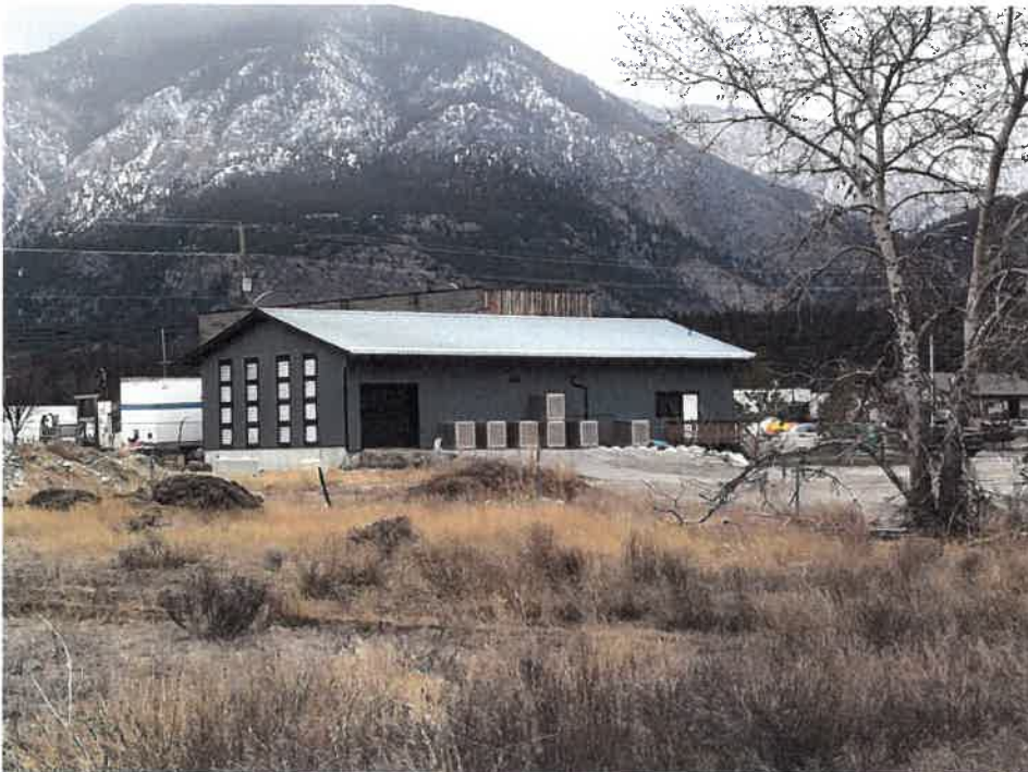
View to northeast from within property toward existing commercial building on property
