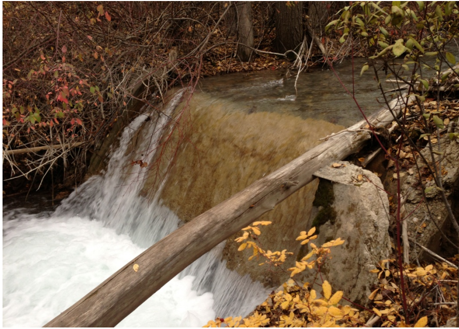
Photo 21. Concrete diversion weir upstream of Windermere Loop Road culvert, Sta. 4+190.
