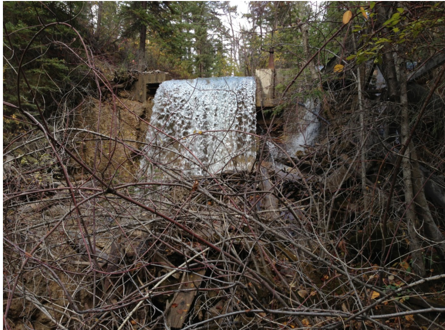
Photo 20. Base of WVGC weir appears vulnerable to undermining erosion, Sta. 4+590. Water on photo right is mostly leakage from intake pipe, but some flow from beneath the weir structure is also visible, which may be a low level outlet.
