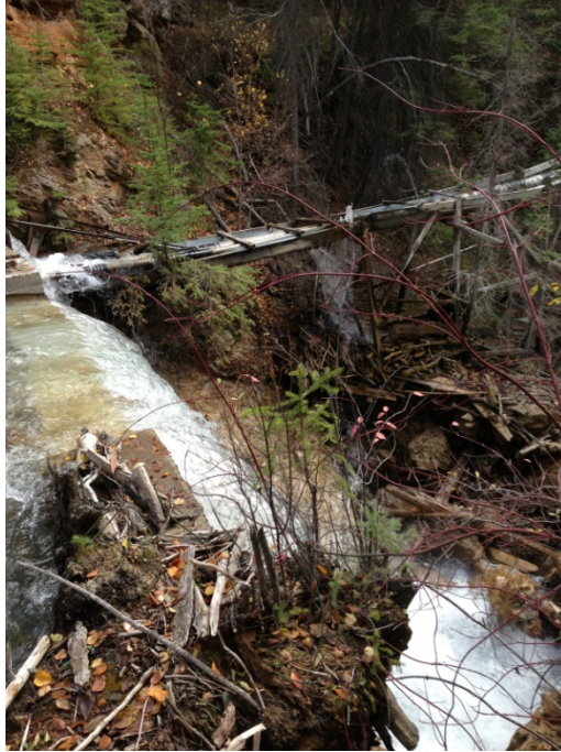
Photo 19. WVGC weir drops 6 – 7 m, Sta. 4+600; diversion pipe is visible in background.
