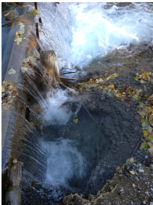
Photo 7. Plunge pool at the base of the Alpine Ranch diversion weir, Sta. 5+600.
