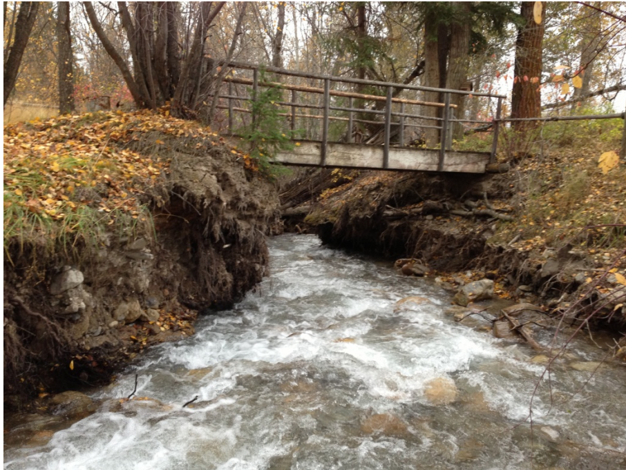
Photo 24. Incised channel downstream of Windermere Loop Road culvert, with undercut banks, Sta. 4+100.
