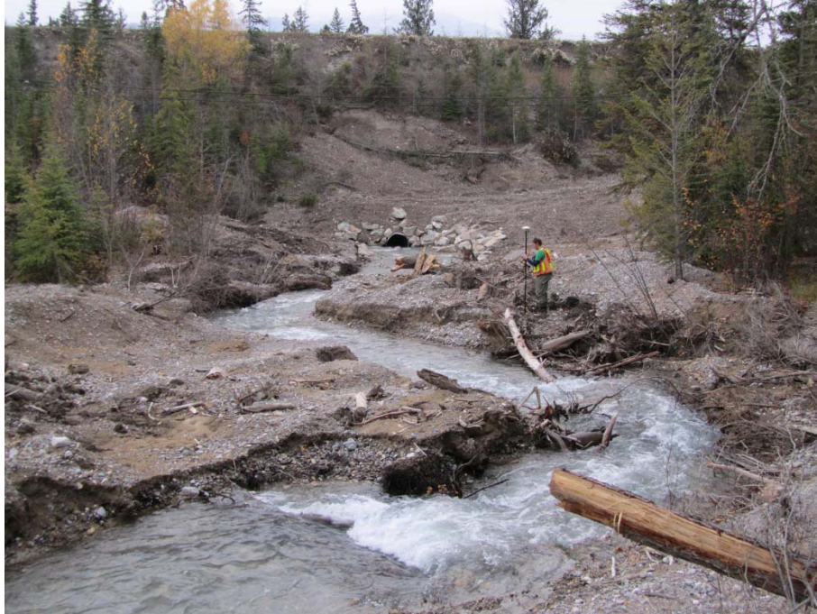
Photo 27. Downstream view of sediment deposition in the reach upstream of Highway 93, Sta. 1+650.
