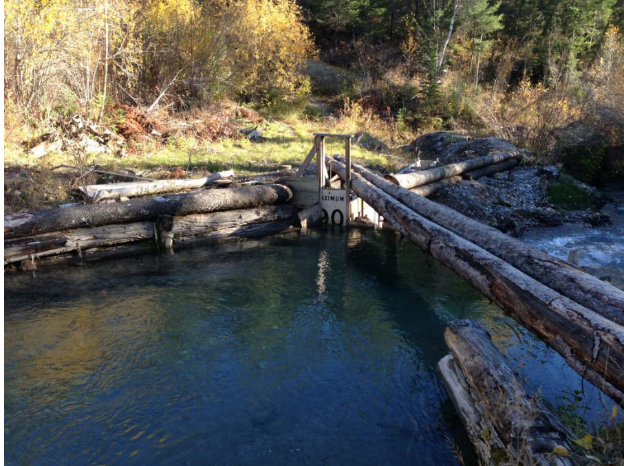
Photo 6. View facing the left bank of the Alpine Ranch diversion weir, Sta. 5+600. The speed limit sign acts as a gate to control flow into the diversion channel.
