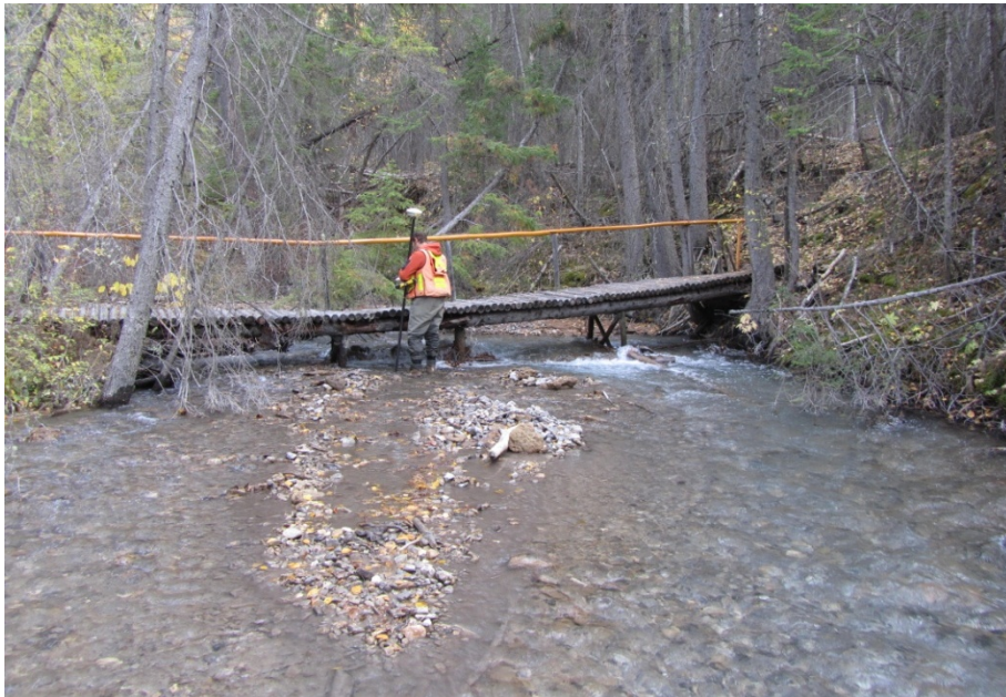
Photo 18. Upstream view showing aggrading bed upstream of WVGC weir, Sta. 4+650. Note buried bridge piers.
