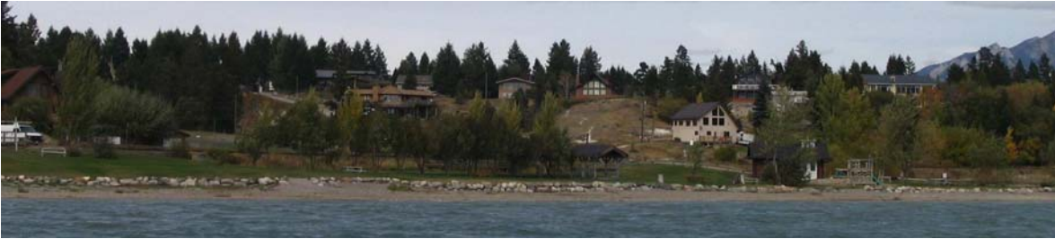
Figure 30. Shoreline modifications along Segment 5 (Columere) include retaining wall, riparian and aquatic vegetation removal and railway. Photo: Leschied Sept 2007.
