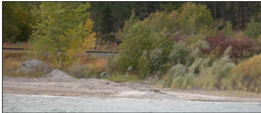
Figure 20. Marion Creek in Segment 7 entering lake through culvert under the railway. Photo: Porto Sept 2007.
