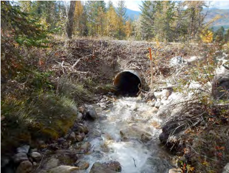
Photo 14: Reach 3. Inlet of culvert (1200 mm) at Fairmont Resort Rd.
