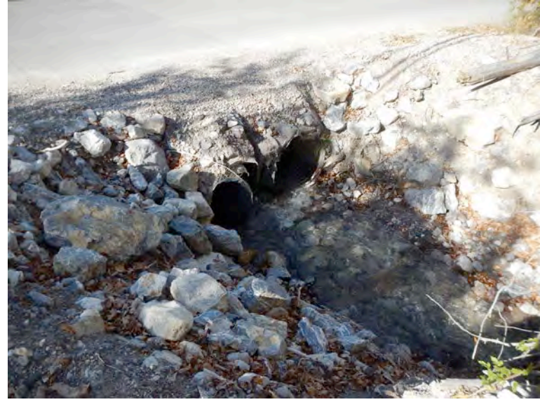
Photo 11: Reach 3. Inlet of culverts (900 mm & 800 mm) at Hot Springs Rd.
