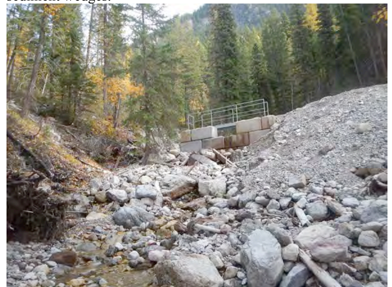
Photo 25: Downstream face of FHSR Water Intake Weir
