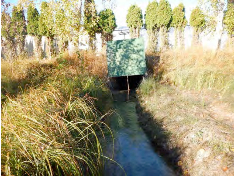
Photo 1: Culvert (1600 mm) and gate at outlet of RDEK Debris Trap (towards Columbia River)
