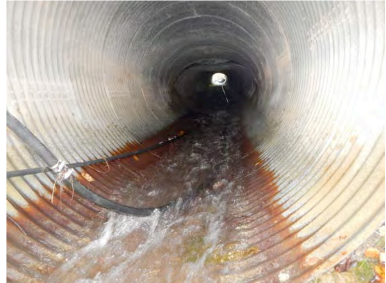
Photo 7: View upstream through Hwy 93/95 Culvert. Note deformation and water lines.
