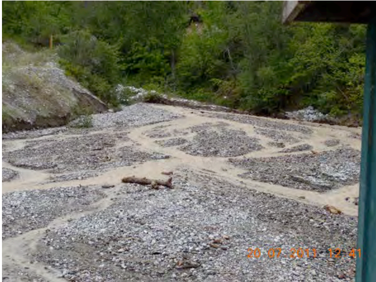
Photo 34: Sediment infilling of Cold Spring Dam reservoir after flood event in 2011 (photo from RDEK)
