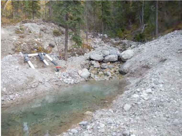
Photo 26: FHSR Water Intake infiltration gallery
