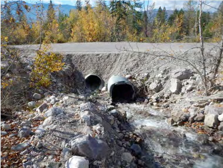
Photo 13: Reach 3. Inlet of culverts (1200 mm & 900 mm) at Fairway Road.
