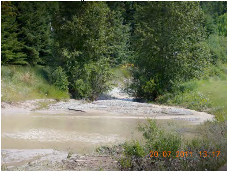
Photo 35: Sediment infilling of lower debris trap on Cold Spring Creek after flood event in 2011 (photo from RDEK)
